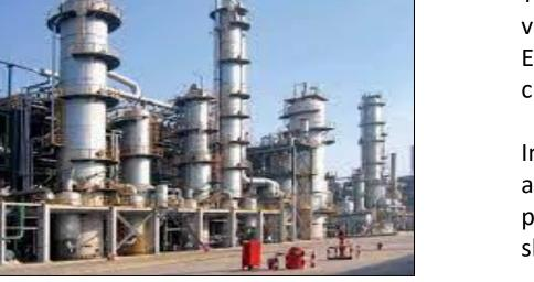
The Vinyl Chloride Column, provides purified vinyl chloride as overhead product and an EDC bottoms product essentially free of vinyl chloride.
